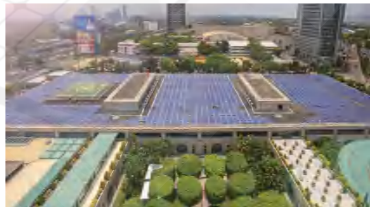
Asian Development Bank Rooftop Project Philippines System Capacity: 571 KW
