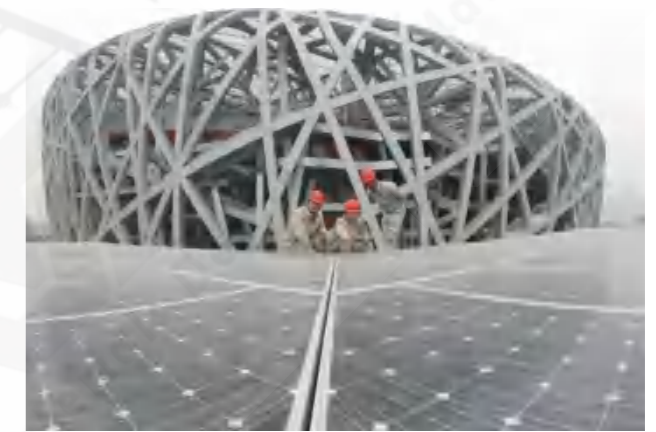
Bird's Nest Stadium BIPV Project China System Capacity: 130 KW
