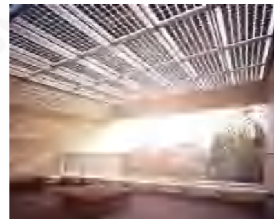
Kowa Elementary School BIPV Project Japan System Capacity: 10 KW
