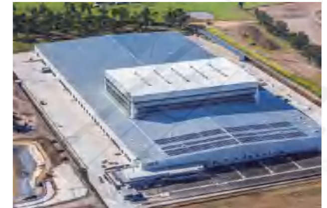
IKEA Rooftop Project Australia System Capacity: 384 KW
